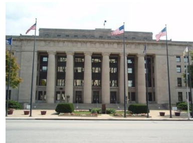
Wyandotte County Courthouse
